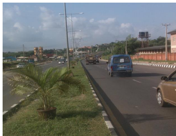
Plate 2: Six (6) lanes road along Abiola way Authors' Field Survey, 2019
