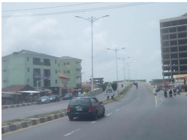
Plate 1: Grade Separation at Ibara, Abeokuta Authors' Field Survey, 2019
