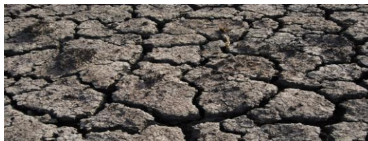
Fig. 1.1 Typical Cracks in Black Cotton Soil of selected areas within Ilaro
