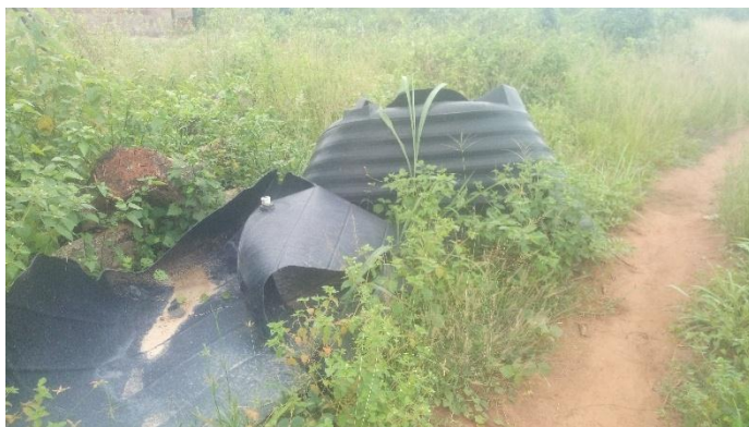
Plate 4: A view of collapsed storex water tank Source: Authors' field survey
